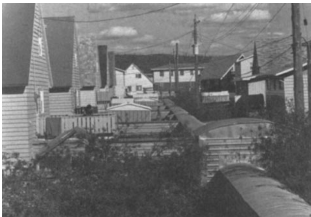
Fig. 6. Utilidor used for servicing houses in Inuvik, Northwest Territories. (Slide 18)
