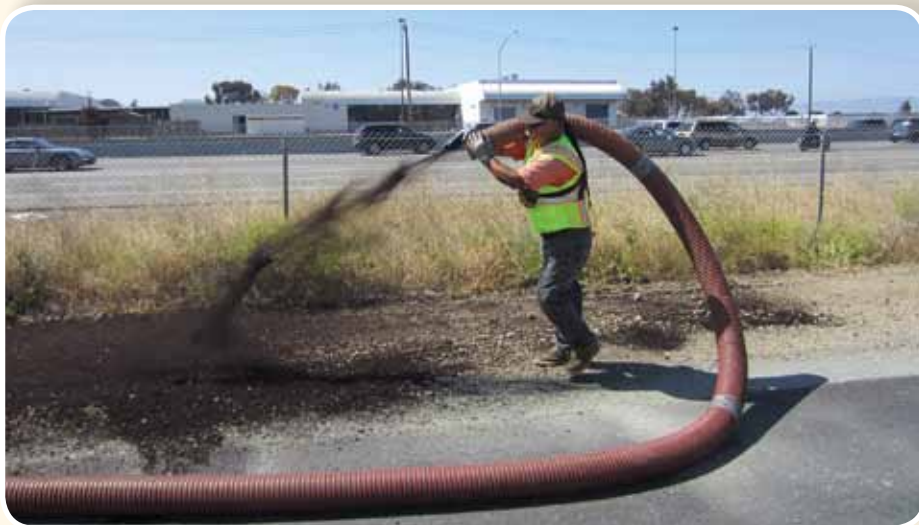
Compost blanket installation. Photo courtesy of San Jose Parks.
