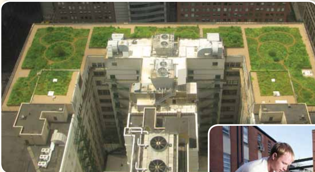
Left: Chicago City Hall green roof. Photo courtesy of Wikipedia/ Tony the Tiger. Bottom: Ed McLean, a landscape supervisor with Appalachian State University's Physical Plant, weeds the green roof on the W. Kerr Scott Hall. Photo by Marie Freeman.
