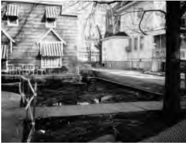
Exhibit 1. Photograph of soil excavation efforts in Joplin, MO. Photo credit Jim Mueller.
