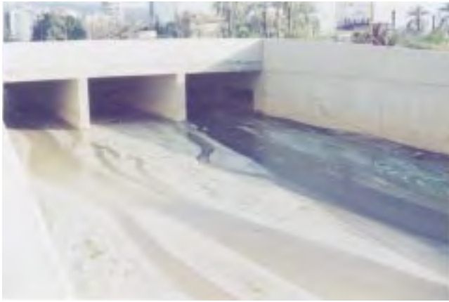
Exhibit 2. Culvert carrying untreated wastewater to an offshore outfall.
