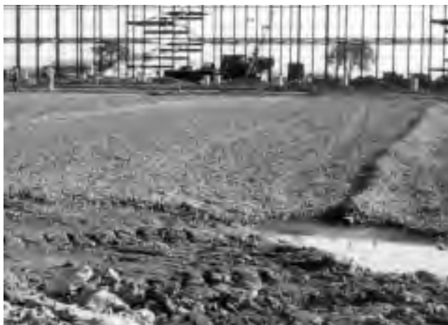
Fig. 1. Installation of gravel blanket during construction in 1959.
